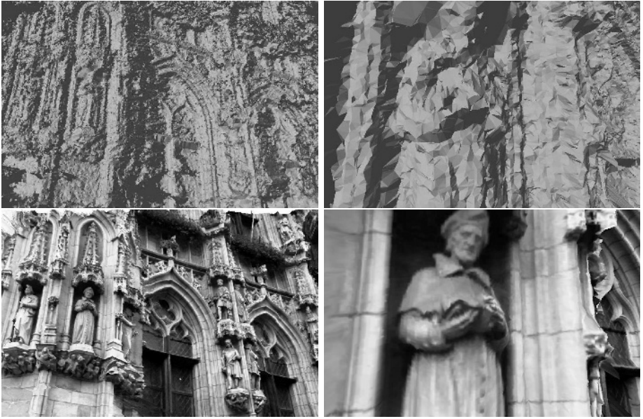
Fig. 4. Untextured and textured views of the reconstructed city hall using the adaptive triangulation method
